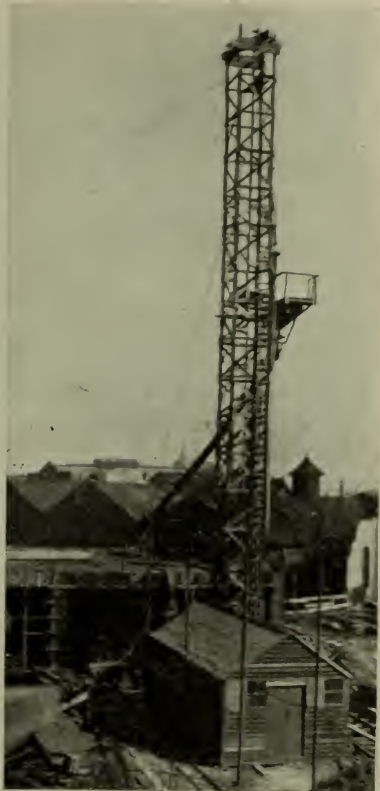
NEW WORKSHOPS FOR THE GAS LIGHT & COKE CO.: CONCRETE CHUTING PLANT.
